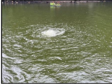
Figure 11: Aeration diffuser not working properly
